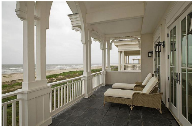
Figure 14 - Porch with columns, brackets & guard
