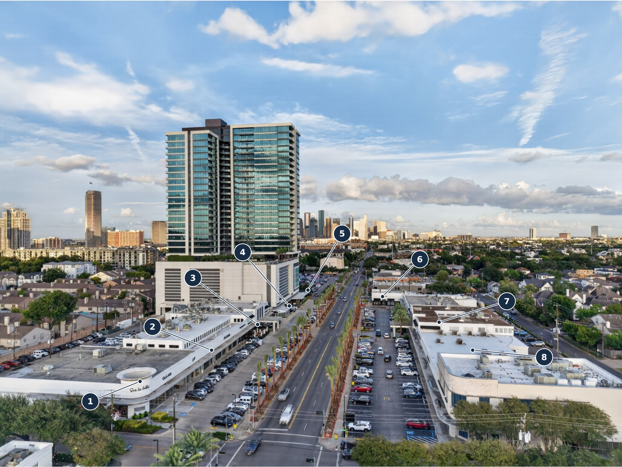
WEST GRAY STREET / VIEW LOOKING EAST
