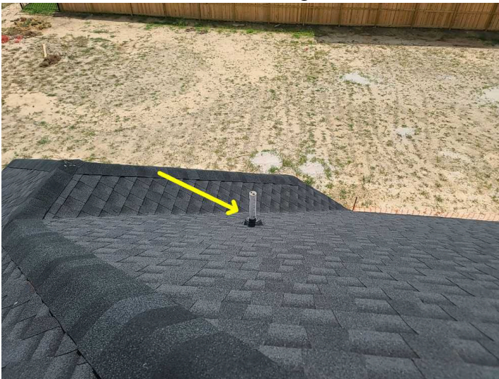
Rubber gasket of drain waste vents have an inverted rubber gasket
