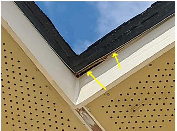
Metal drip edge is lifted/ bent at the East roof edge above back patio.
