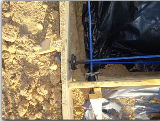
The front form boards are incomplete and final punch-out has not been performed.
