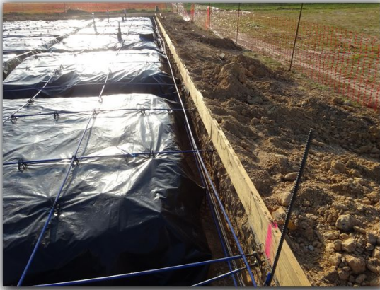
The front form boards are incomplete and final punch-out has not been performed.
