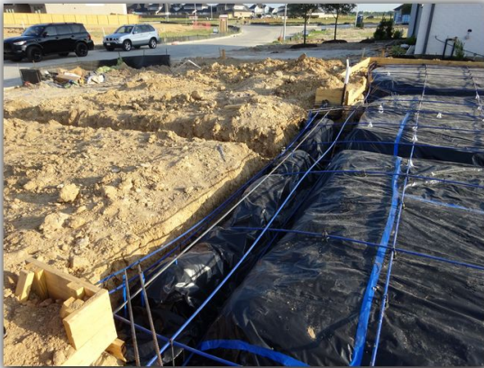
The front form boards are incomplete and final punch-out has not been performed.
