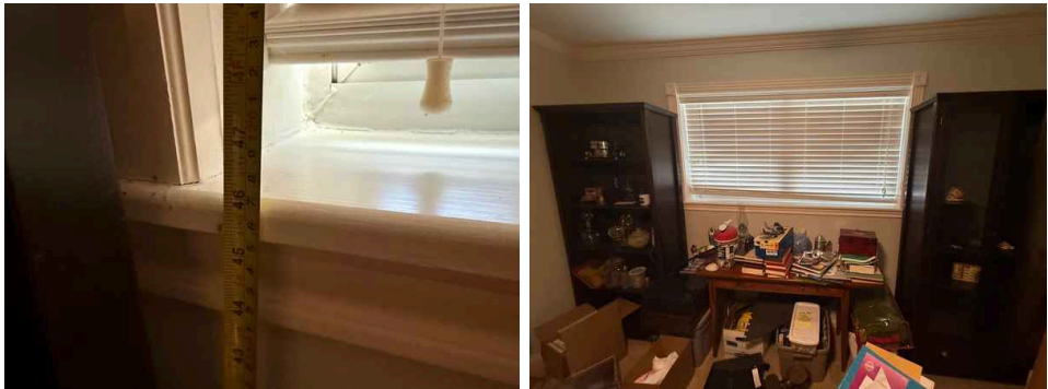
Figure R310.1 EMERGENCY ESCAPE AND RESCUE WINDOW
