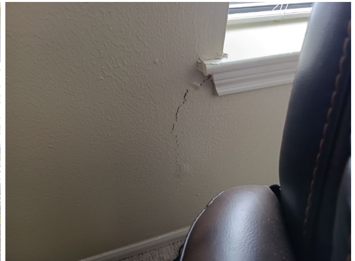
Stress crack
