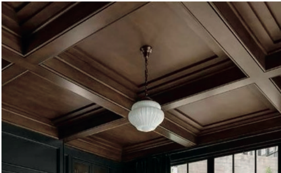
Wood Coffered Ceiling
