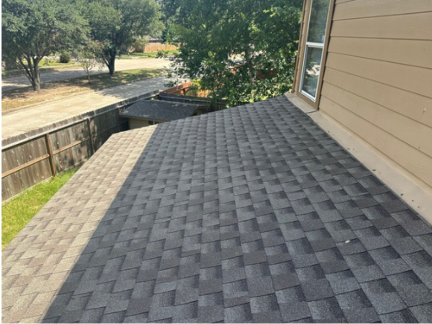
Rear patio cover. Excellent condition
