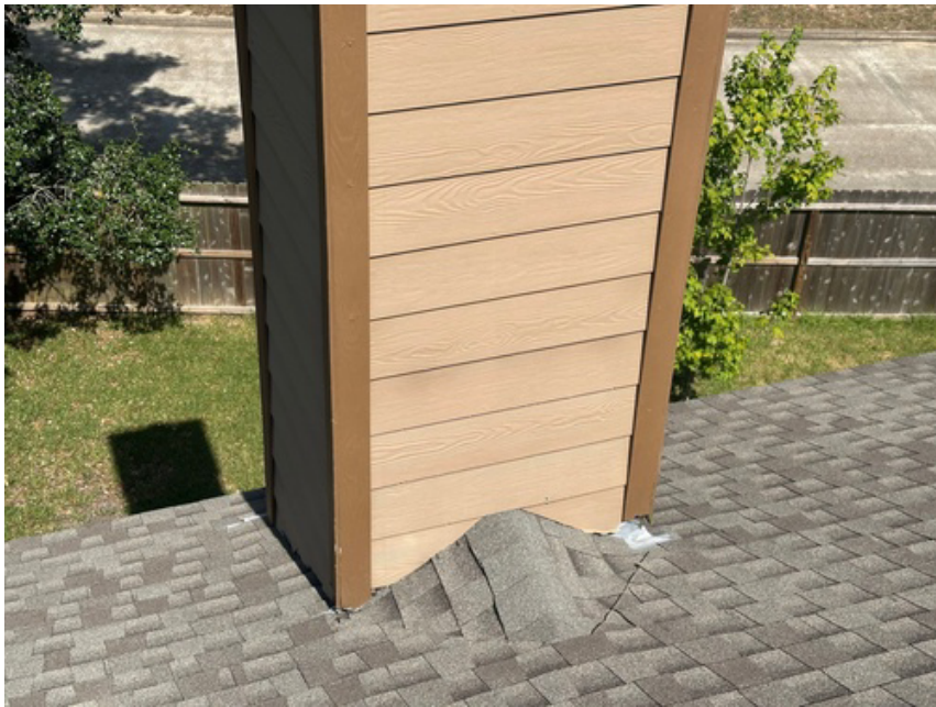
Chimney cricket. Excellent condition
