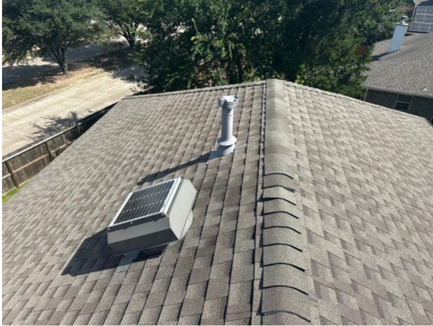
Ridge Vent functioning properly. Excellent condition
