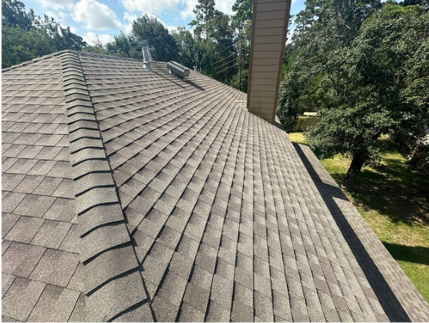
Rear main slope and accessories. Excellent condition.
