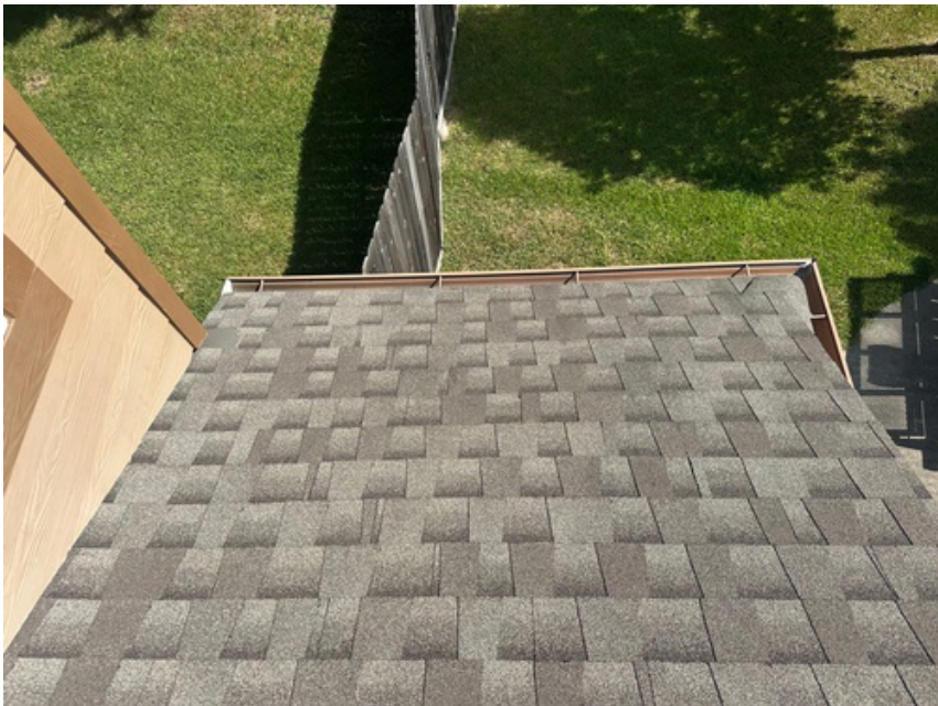
Side slope. Excellent condition
