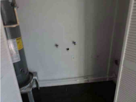
Unit A Utility Room
