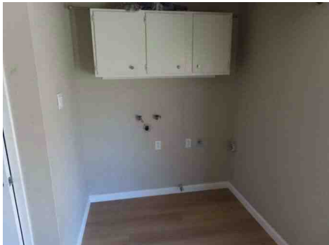
Unit B Utility Room
