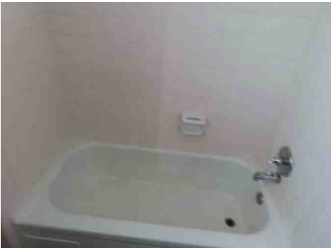
Unit A Bathroom 2 Detail
