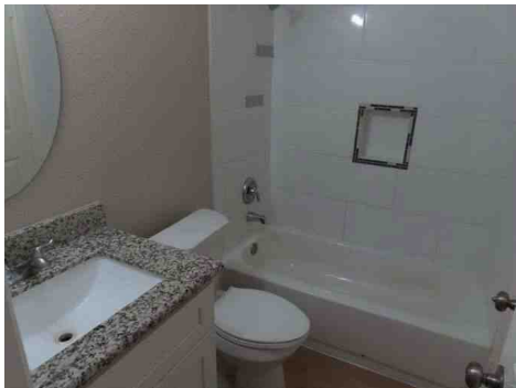
Unit B Bathroom
