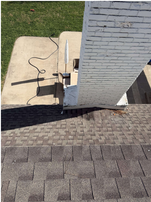
Chimney Flashing in good condition
