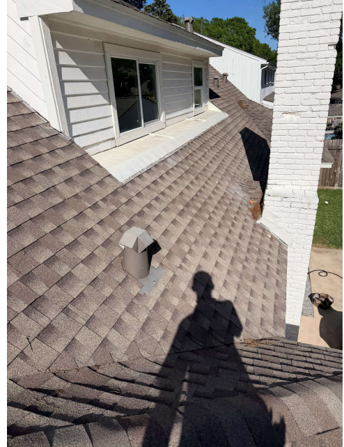
Metal vents and products in good condition
