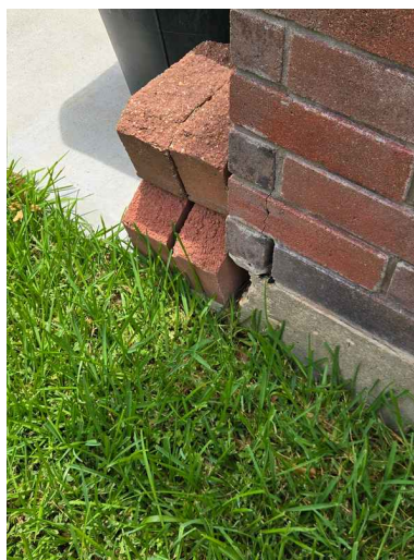
Corner Pop/ "Wedge Crack" Example
