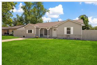
Another front view displaying the newly installed windows, fresh paint, new roof and new privacy fence
