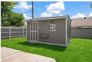
Storage shed freshly painted with new roof. Grass has been digitally enhanced for photos.
