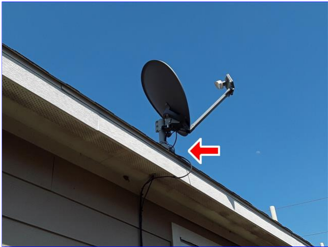
C. Item 1 (Picture) right side of the roof
