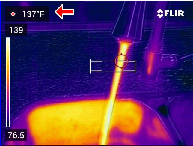
A. Item 1 (Picture) hot water temperature
