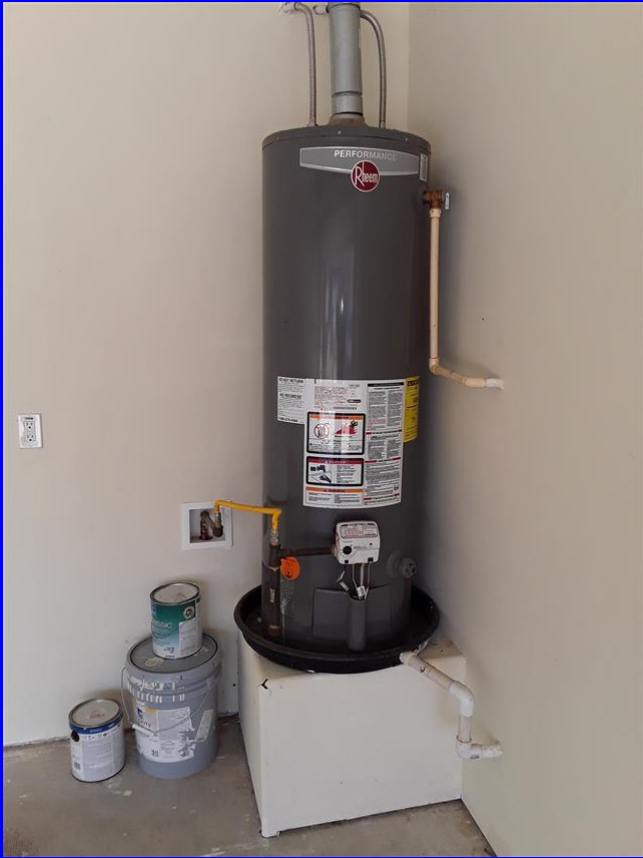
Rheem 40 gallon gas water heater located in the garage
