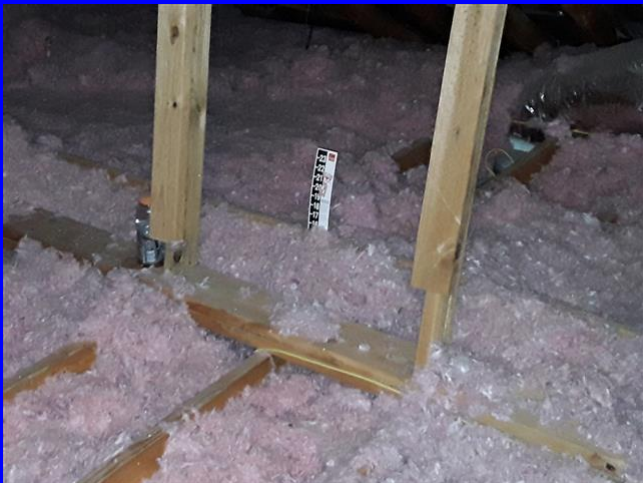
approximately 12 inches of insulation in the attic
