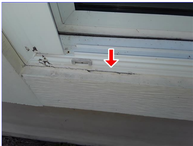
H. Item 2 (Picture) seal all windows where needed
