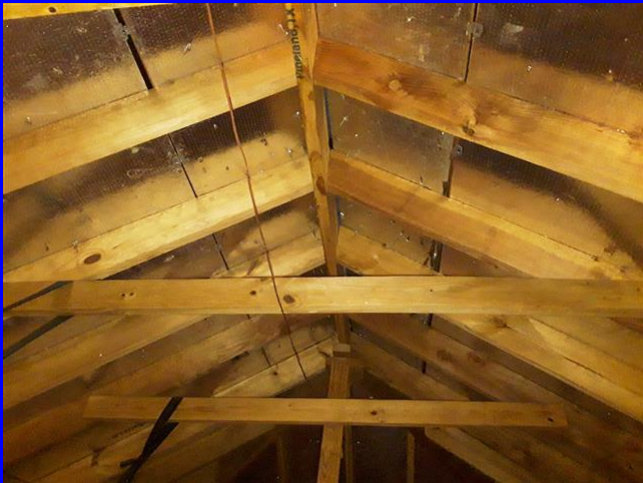
Stick built roof structure with radiant barrier decking
