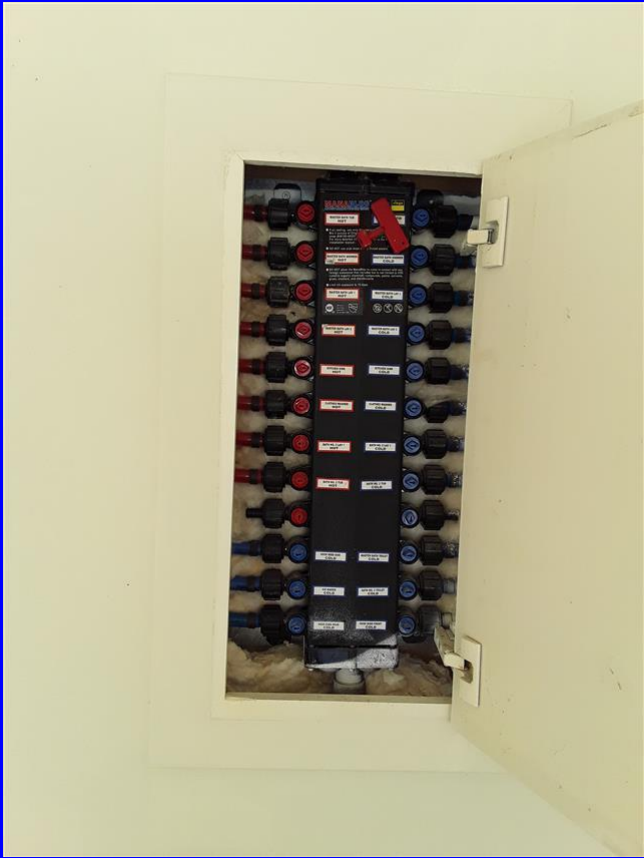
PEX water distribution manifold located inside the garage on the rear wall
