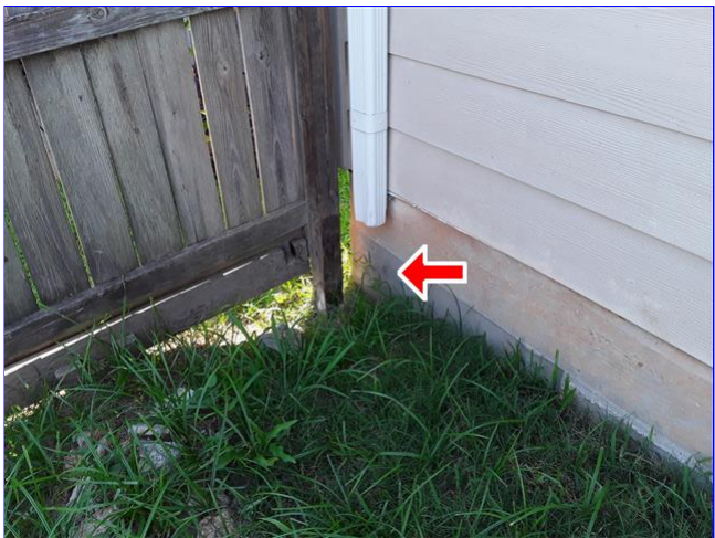
B. Item 2 (Picture) rear right corner of the foundation
