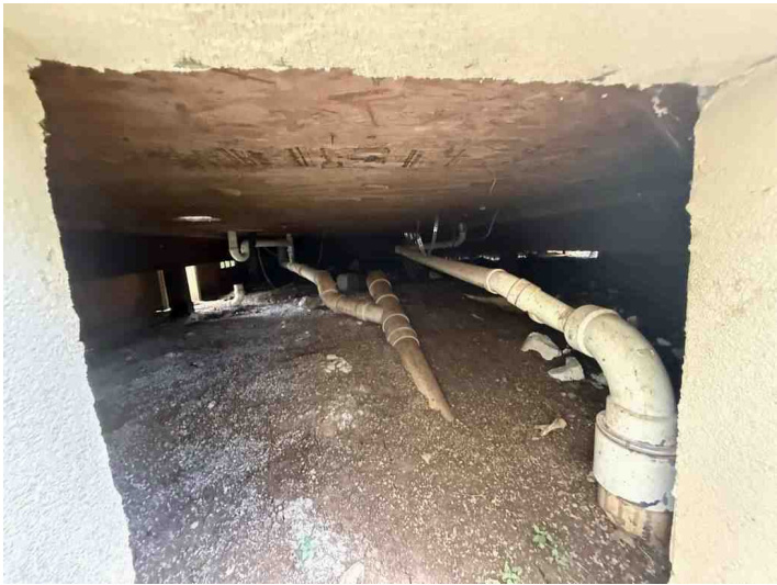
Crawlspace Main House
