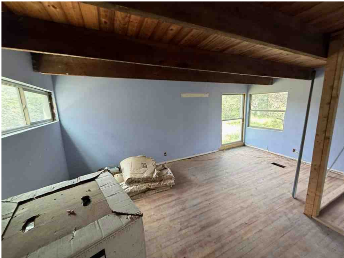
Bedroom 2 Main House
