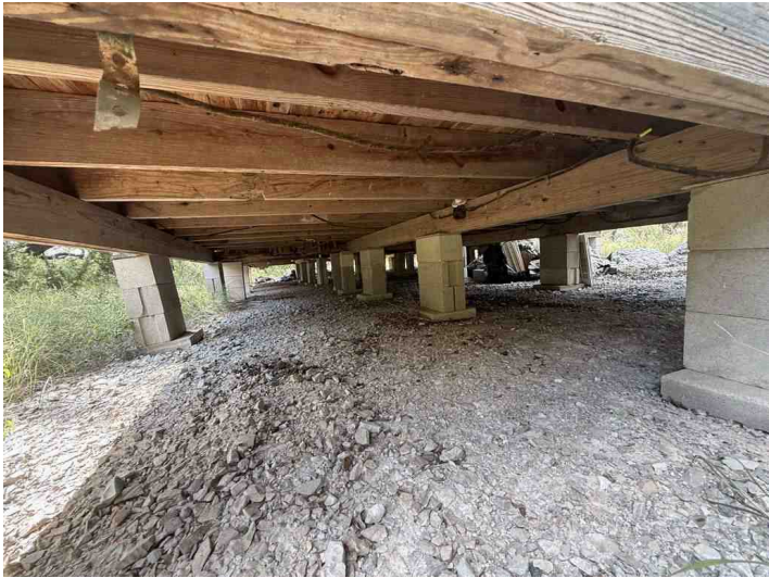
Crawlspace Second House
