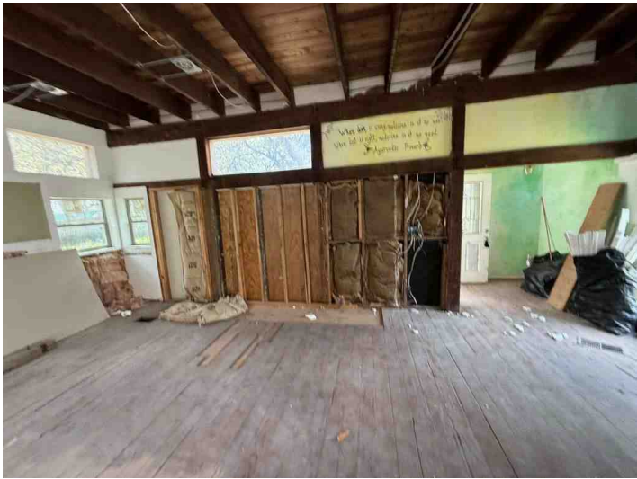
Living Room Main House
