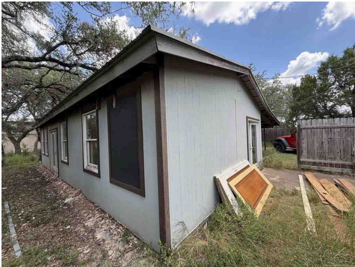
Rear View Casita
