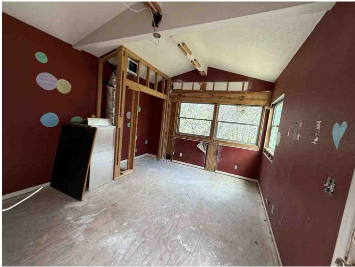
Bedroom 3 Main House
