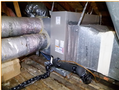
Evaporator coil
