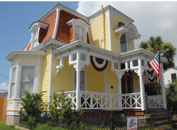
DARLING’S BIRDCAGE The two pictures above of 1301 Broadway were taken on March 31, 2019 before the home was extensively damaged when the water pipes burst during the winter storm in February 2021. On the opposite page is an aerial photo taken of Galveston in 1930 that features the area between 13th Street and 14th Street, and Broadway and Sealy. The house is located in the middle part of the picture at the bottom. It’s third-story mansard roof (now gone) is said to have been the first of its kind on the island and resulted in the home becoming quite a novelty, coming to be known as Darling’s Birdcage.
