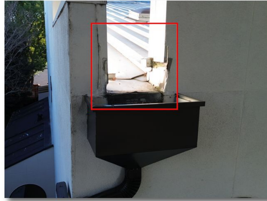
1- 2.8 Seal scupper drain
