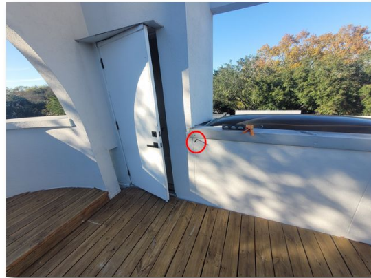
6- 1.2 Test Location H - Soft substrate encountered
