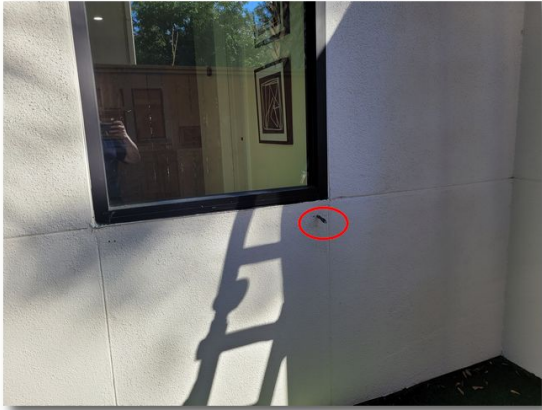
2- 1.7 Test Location H - Soft substrate encountered
