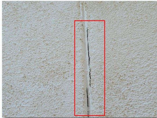
4- 3.8 Control joint crack
