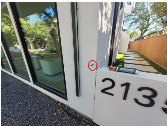
1- 1.3 Test Location K - Soft substrate encountered
