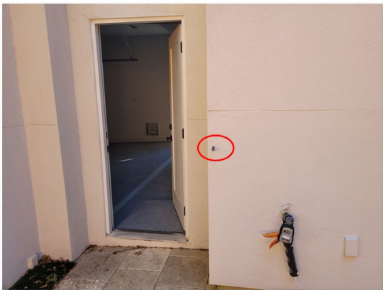
4- 1.3 Test Location C - Soft substrate encountered
