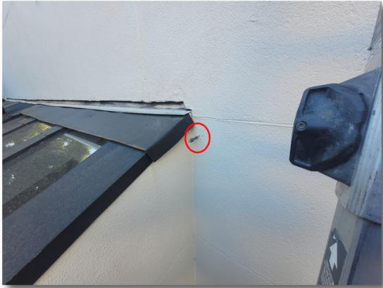
5- 1.5 Test Location M - Soft substrate encountered
