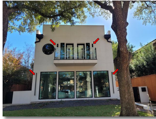
1- 2.6 Seal top mount fasteners on balcony
