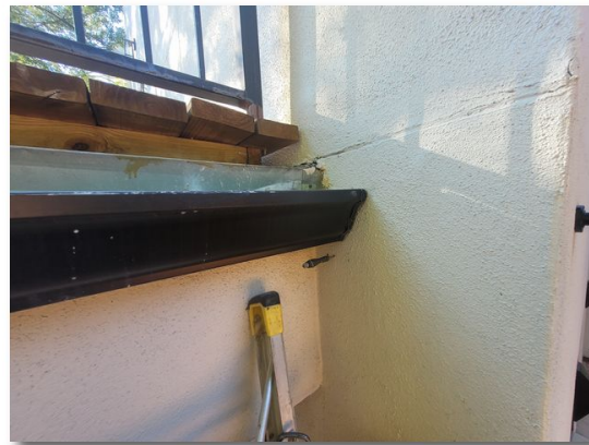
4- 1.4 Test Location D - Soft substrate encountered
