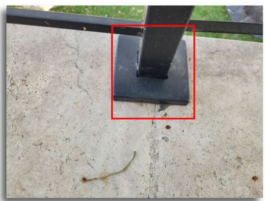
1- 2.6 Seal top mount fasteners on balcony
