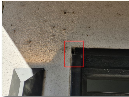
3- 1.4 Seal void at top left corner of garage
