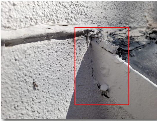
2- 2.7 Seal roof / wall intersections
