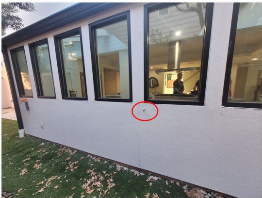
5- 1.3 Test Location F - Soft substrate encountered
