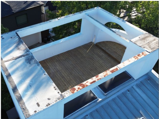
G- 4.1 Seal cap flashing around roof line
