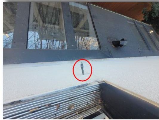
5- 1.6 Test Location O - Soft substrate encountered
