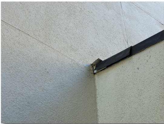
4- 2.7 Seal roof / wall intersection
