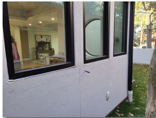
5- 1.4 Test Location I - Soft substrate encountered
