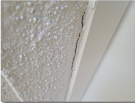
4- 2.7 Seal roof / wall intersection
