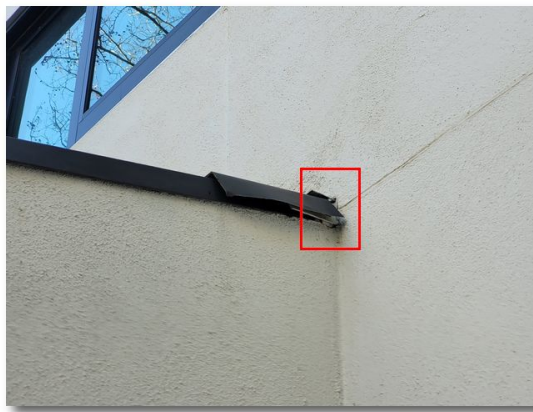
5- 2.4 Seal roof / wall intersection
