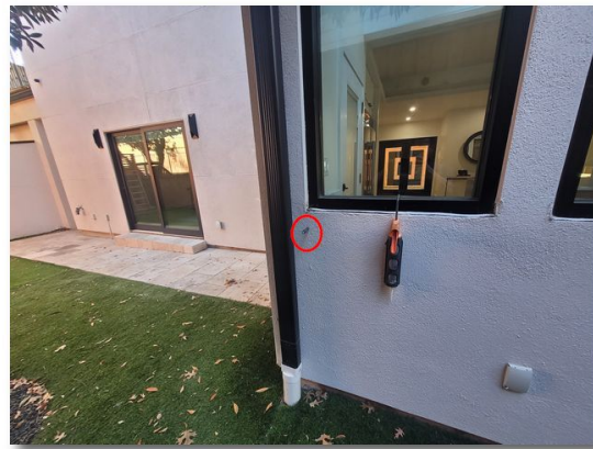
5- 1.4 Test Location I - Soft substrate encountered
