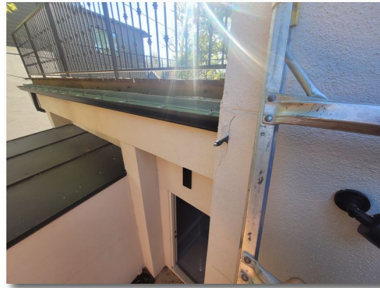
4- 1.4 Test Location D - Soft substrate encountered
