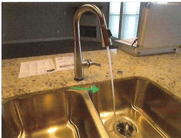
water being run during inspection
