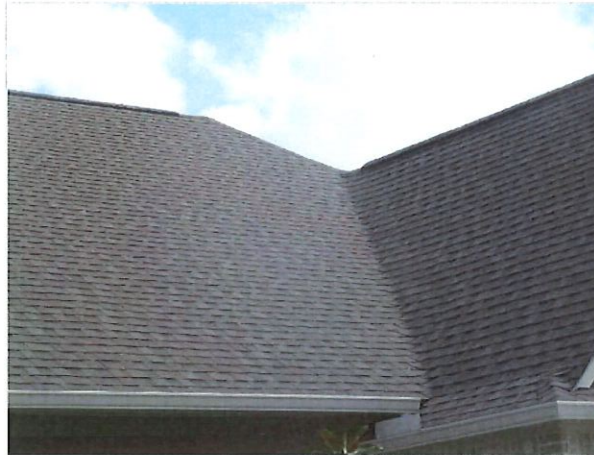
view of roof
