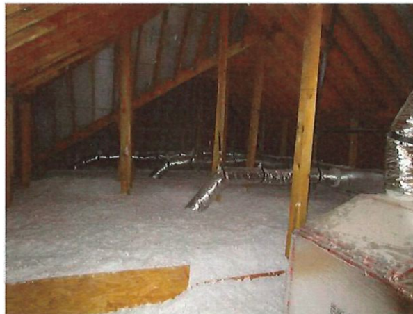
limited access in attic
