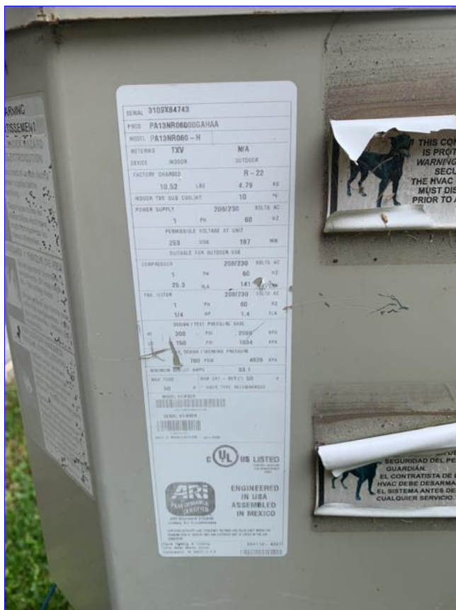
B. Item 1(Picture) AC service tag
