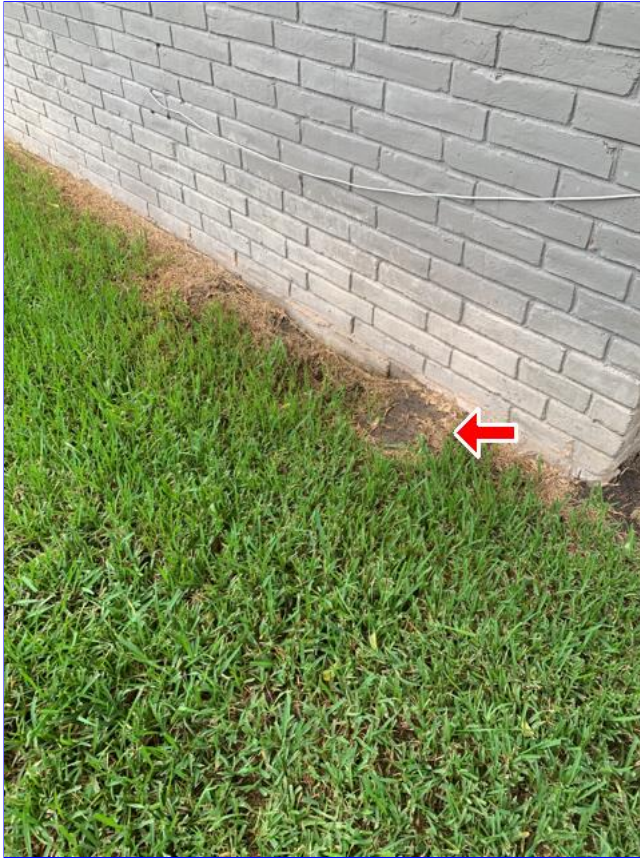
B. Item 2(Picture) Drainage swales at rear and sides of home appears to have low spots.
