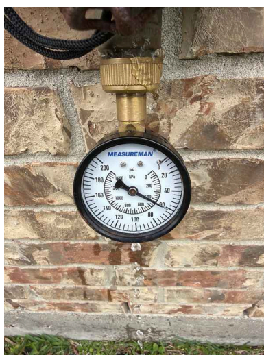
Location of Main Water Supply Valve: RIGHT FRONT CORNER
