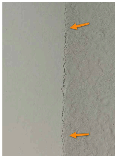
2nd Floor Bathroom #1
