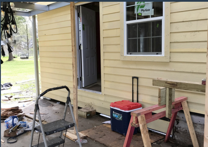
New Siding installed in 2018 and painted
