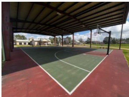
Covered Basketball Court with Full-sized Basketball Hoops and Benches
