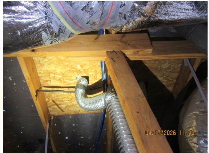
Prior repairs to the roofing material and/or flashing were observed in one or more locations.
