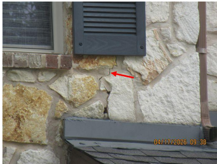
Mortar crack
