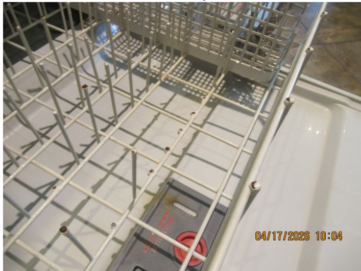
Observed rust on Dishwasher trays
