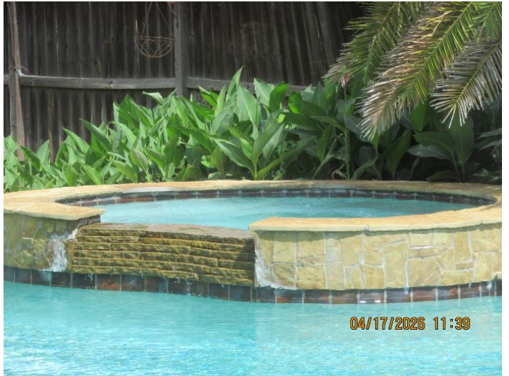
Spa Blower Operational
