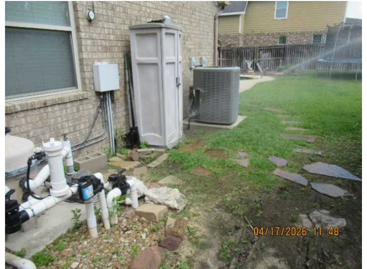
One or more sprinkler heads were in need or adjustment to not spray structure, driveways or other areas.
