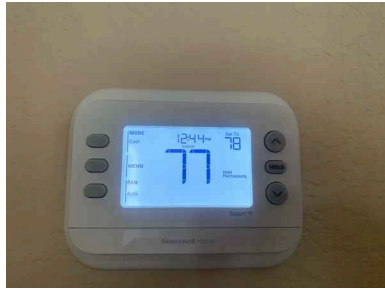
Unit 2- 2nd Floor : Photo of evaporator data plate, Photos of thermostat upon arrival and departure, Photo of vent temperature, Photo of condenser data plate, Photo of condenser, Thermal image of cool air at vent, Photo of return air temperature Delta T Result: 24 Degrees F
