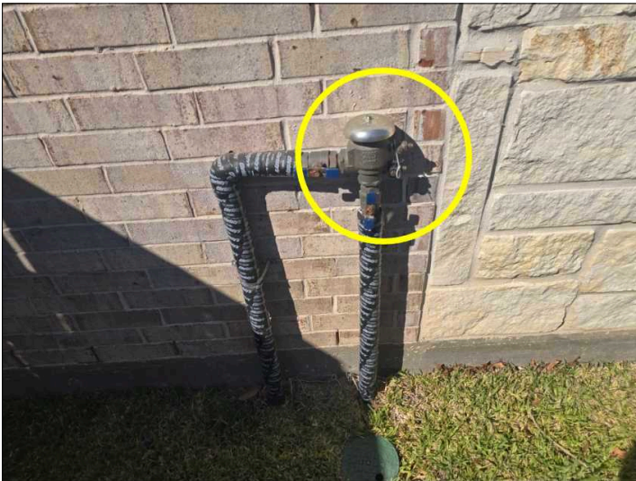
NOTE: Backflow preventer should be protected from weather during winter months.
