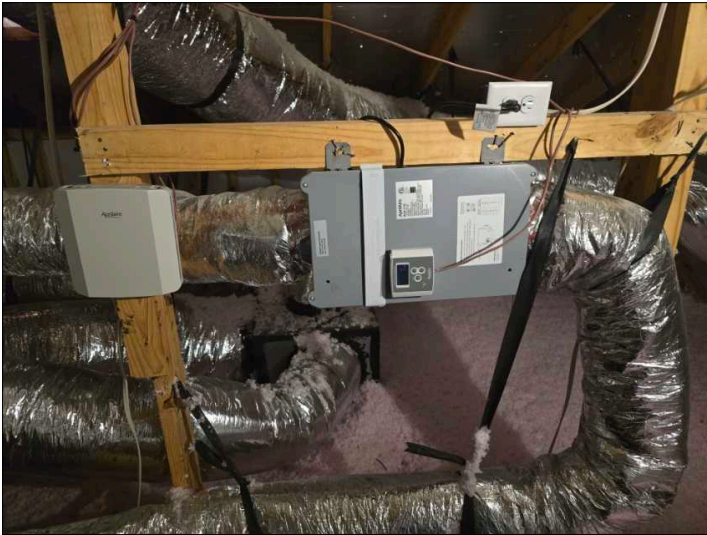
Fresh air intake system present and appears functional. Clean internal filter annually.
