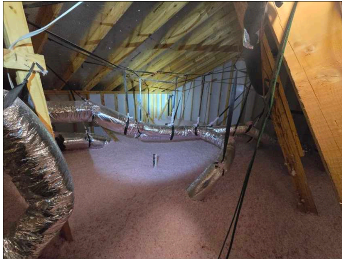
Insulation type(s): Blown fiberglass - newer style
