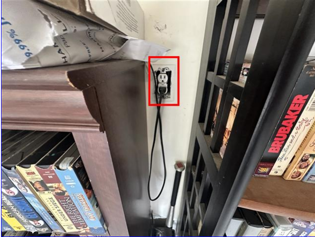
B. Item 5(Picture) garage
