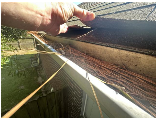
C. Item 19(Picture) left side
