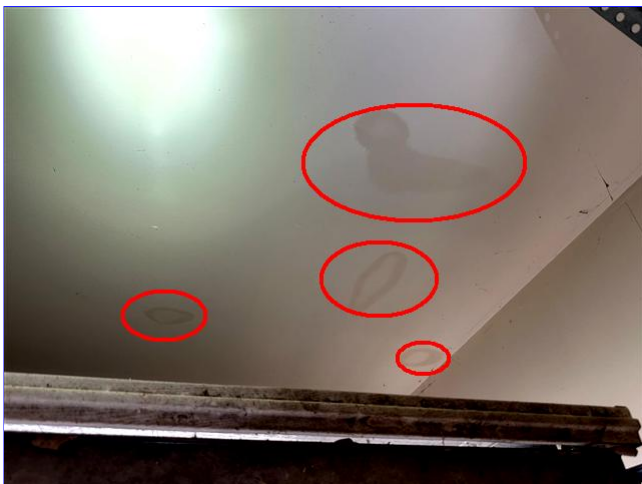
F. Item 3(Picture) garage
