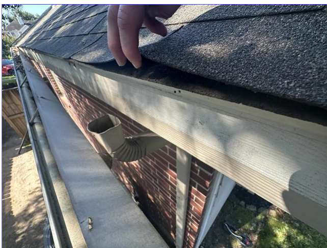
C. Item 18(Picture) right side
