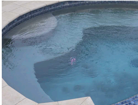
The spa light was operational at the time of the inspection.
