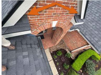
Missing counterflashing
