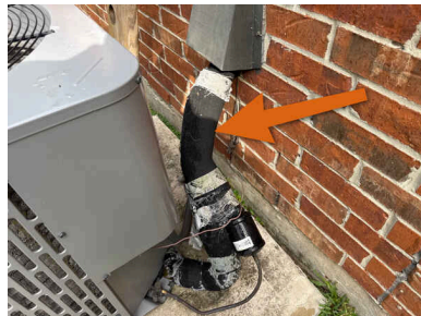
Deteriorated insulation
