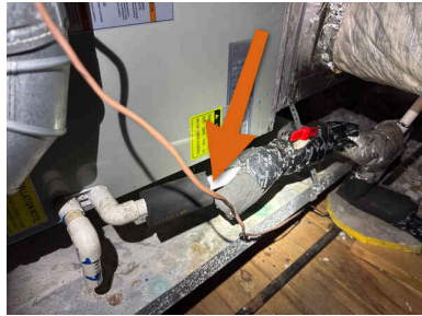
Damaged insulation
