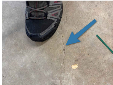
Shrinkage cracks
