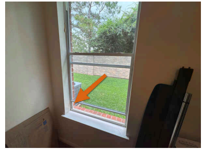
Stuck/separated window balances
