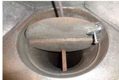
Example of a damper with clamp.
