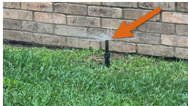
Damaged sprinkler head
