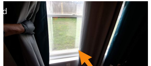
Left window in primary bedroom
