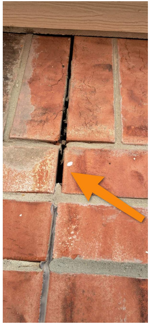
2nd expansion joint on right side
