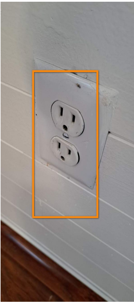
Hall outside of laundry room
