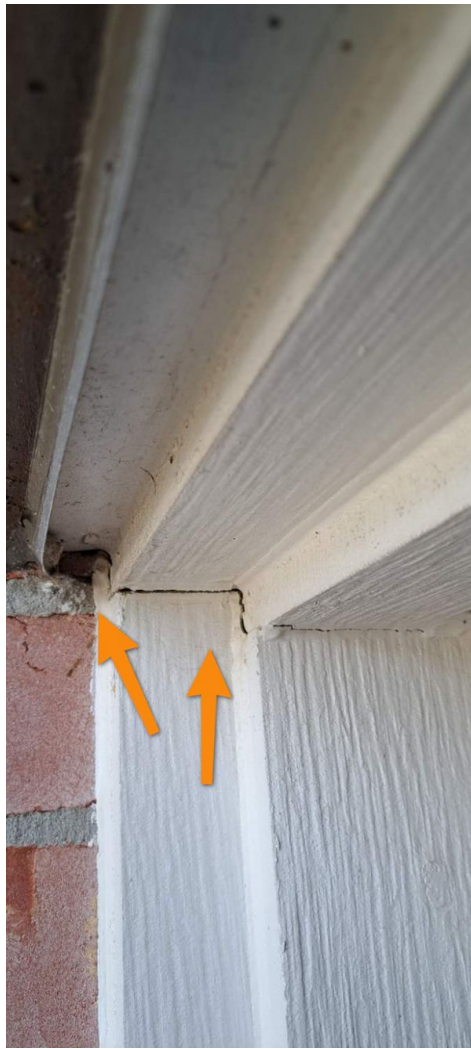
Upper left end at garage opening
