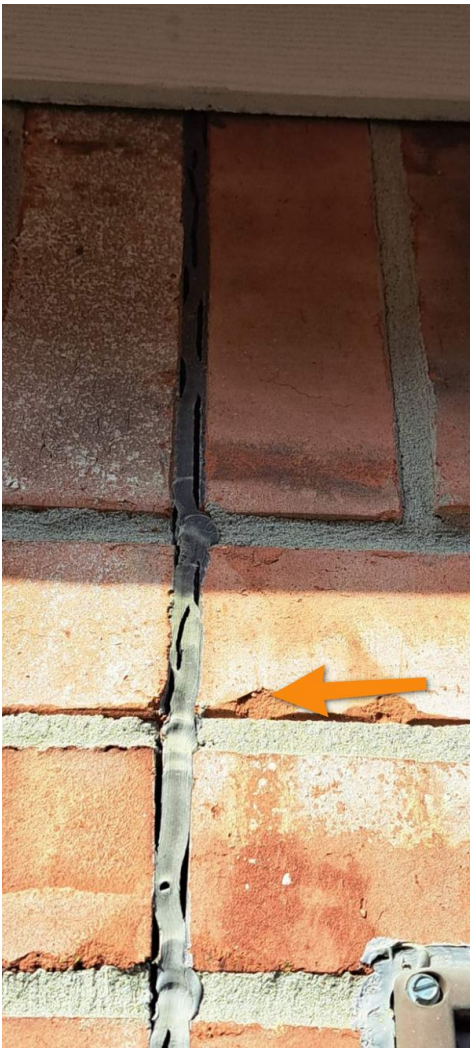
Left side at 1st expansion joint
