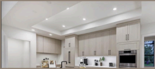
Example of drop ceiling potentially over the cabinets so they appear to go all the way up and eliminate a few feet of space.
