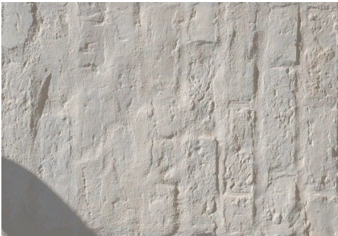
Exterior Brick Slurry
