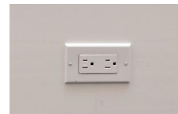
Outlets in baseboards
