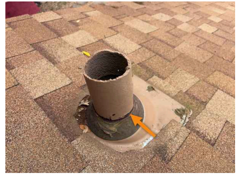
Cast iron drain present
