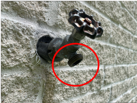
Right: Back flow preventer recommended
