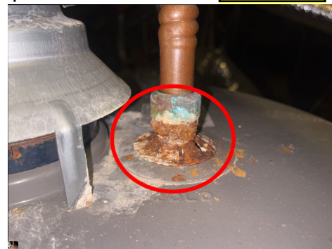
Corroded fitting
