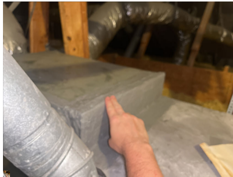
Attic: Evaporating coils sealed/unable to view coils
