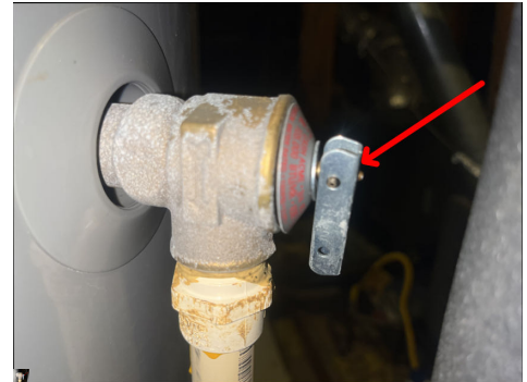
FYI: Test IPR Valve yearly
