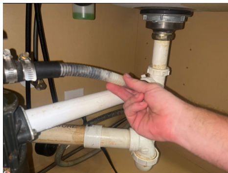
No high-loop or air gap
