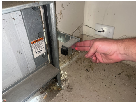
Photo eye sensor more than 6" off ground
