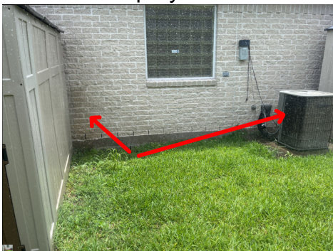
Zone 2: Sprayed structure, condenser
