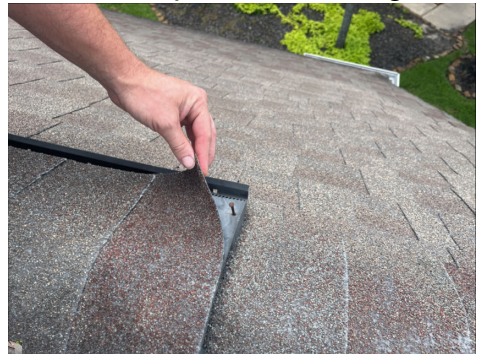
Right front ridge: Loose/uplifted shingle
