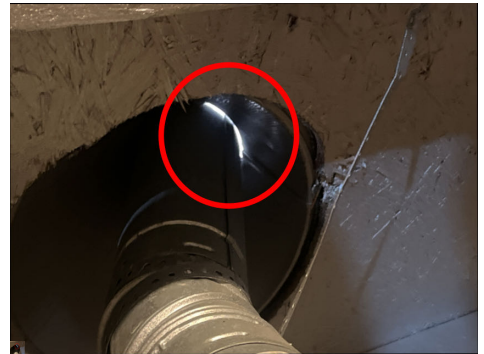
Daylight at roof protrusions
