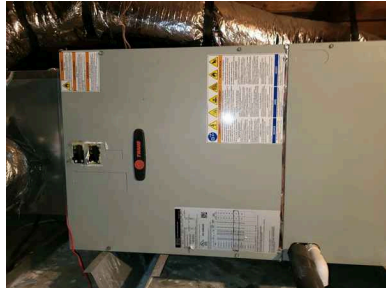
Trane Electric Furnace
