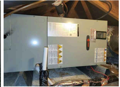
Trane Electric Furnace
