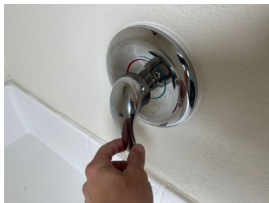
Master Bathroom tub
