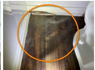
2nd Floor Hall Bathroom right of tub
