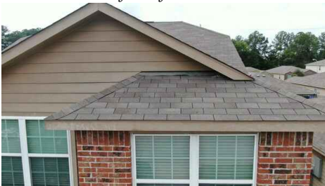
General View Of Roof:
