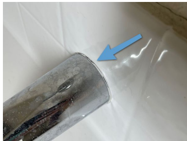
Master Bathroom tub
