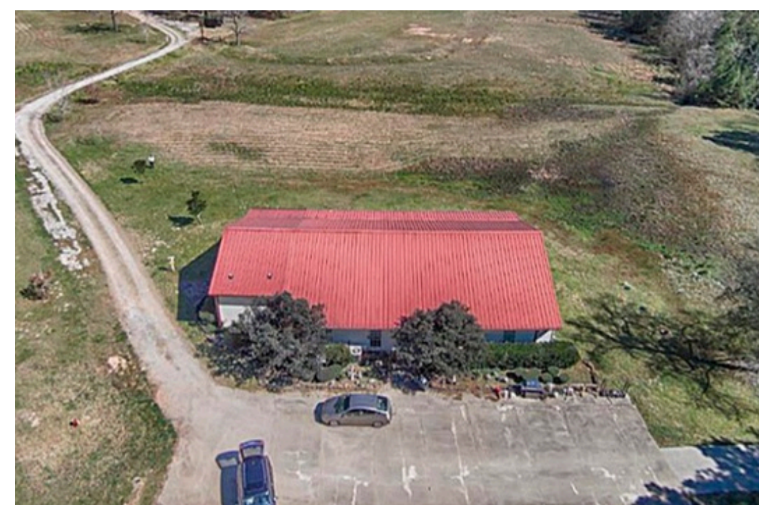
Roads, pathways, bridges and driveways throughout for connectivity
