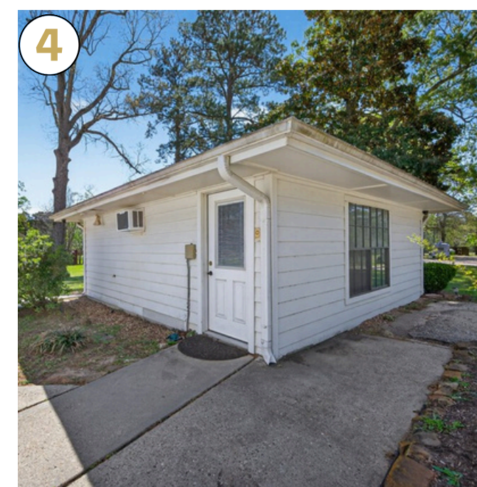
4 Building 4 404 SF Office or private room. Irrigation & Tech room.
