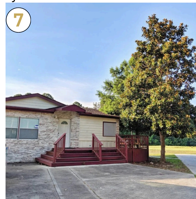
7 Building 7 renovated: 2019 | 2,250 SF cabin. Offices or dormitory
