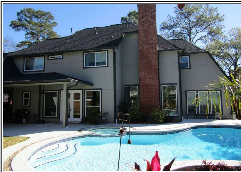
REAR OF SUBJECT PROPERTY
