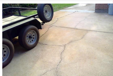
K. Item 1 (Picture) Driveway
