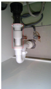
B. Item 1 (Picture) Master bathroom: Drain line for right sink/vanity fixture
