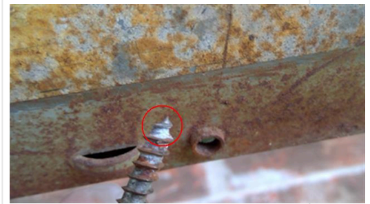
A. Item 3 (Picture) Sharp piercing screw
