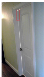
G. Item 7 (Picture) Guest bathroom door
