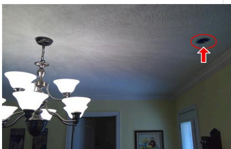
B. Item 4 (Picture) Dining area
