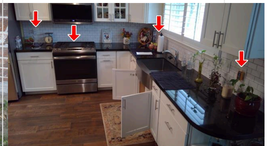
B. Item 3 (Picture) Kitchen GFCI/Oven
