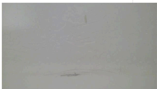
F. Item 7 (Picture) Guest bathroom
