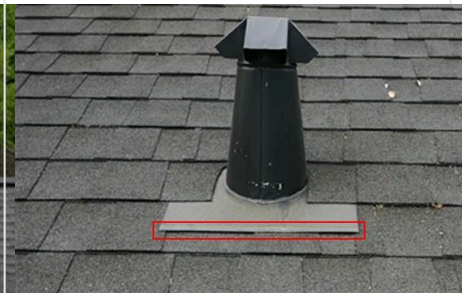
C. Item 5 (Picture) Raised flashing for roof vent
