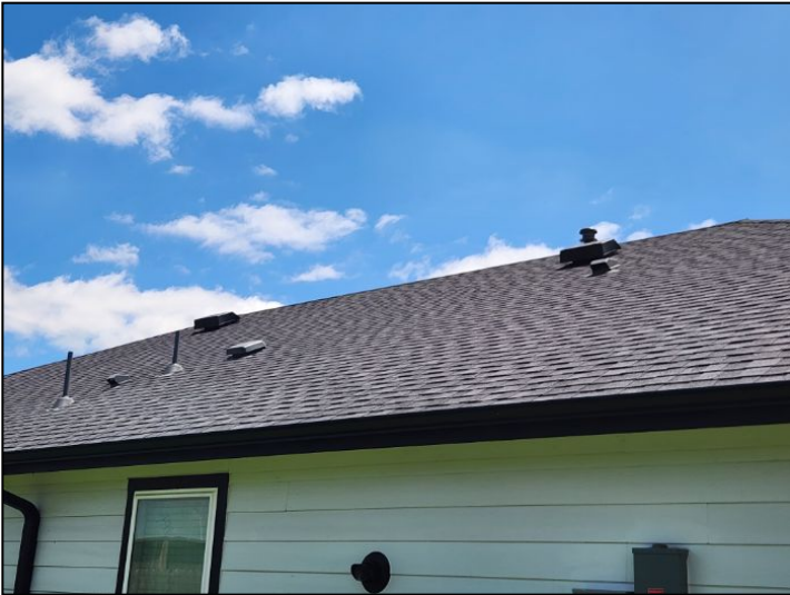
ROOF COVERING; LEFT
