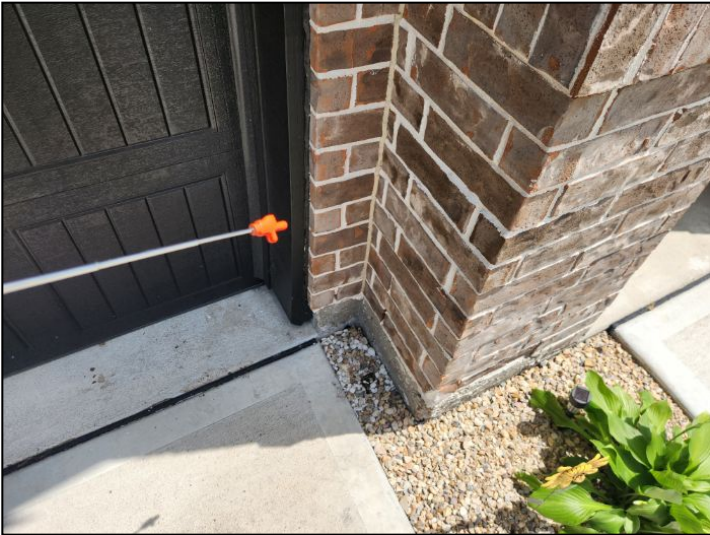
SEAL DETERIORATION
