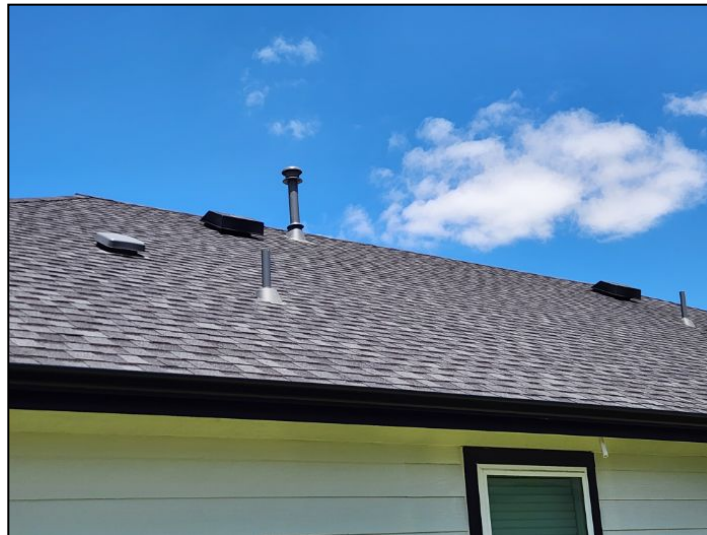
ROOF COVERING; FRONT RIGHT
