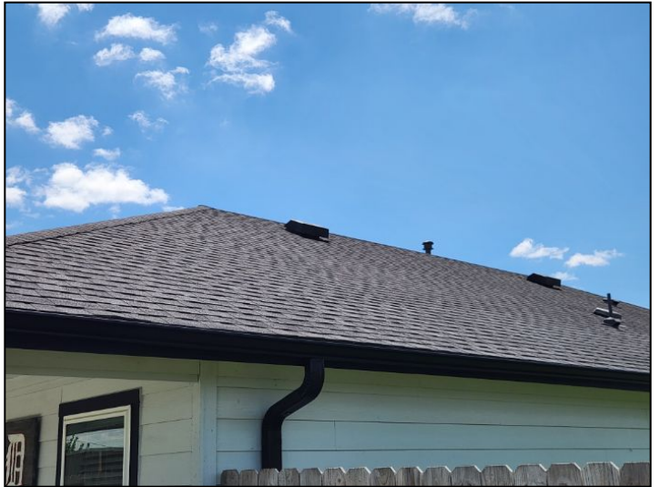
ROOF COVERING; BACK LEFT
