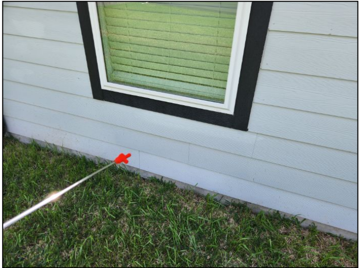
SEAL DETERIORATION
