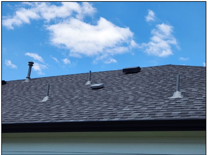
ROOF COVERING; BACK RIGHT
