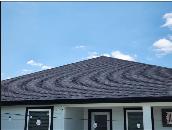
ROOF COVERING; BACK
