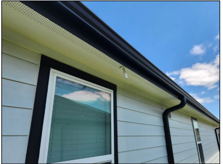
EVAPORATOR SECONDARY DRAIN PIPE ROUTED HERE
