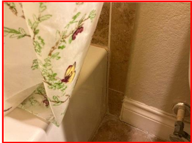
Deteriorated Caulk
