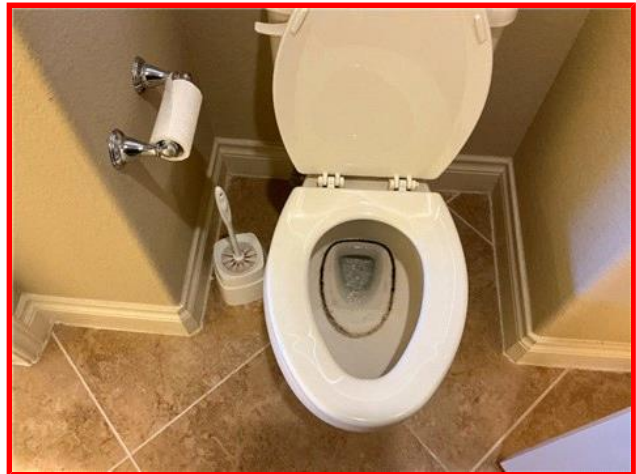
Toilet Seat Loose in Jack and Jill Bathroom
