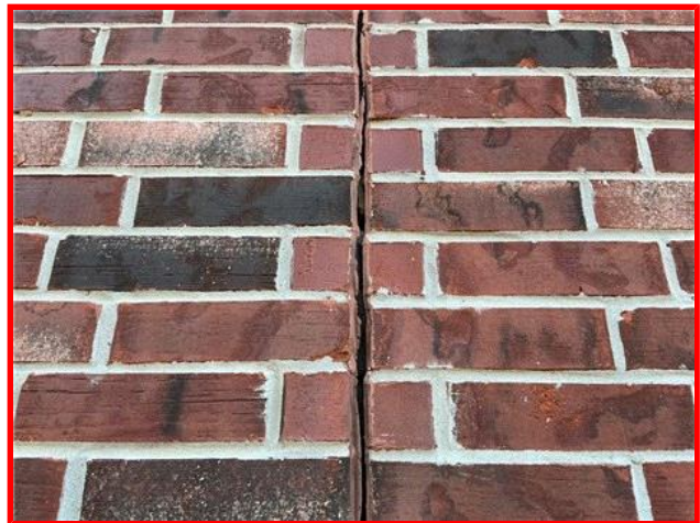
Missing Mortar at Left Expansion Joint
