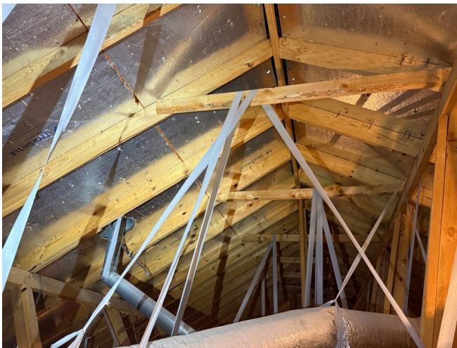
Overview of the attic framing along the main roof ridge
