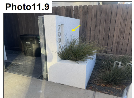
Privacy wall is CMU construction. This is a proper detail.
