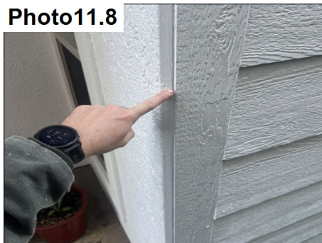
Siding transitions are sealed. Always maintain sealants.
