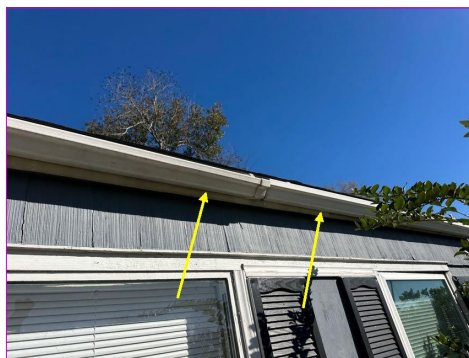
Gutters and downspouts were fabricated from vinyl.
