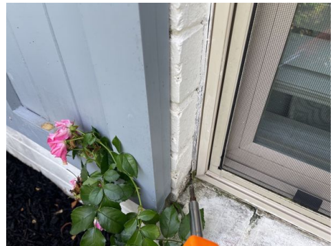
Deteriorated sealants.
