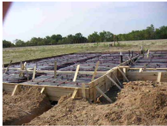
an overview of a post-tensioned slab-on-ground foundation ready for concrete
