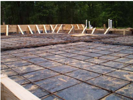
reinforcing steel in field area of a slab-on-ground foundation
