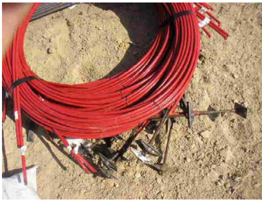
this is a bundle of post-tensioning cables as they are delivered to the site
