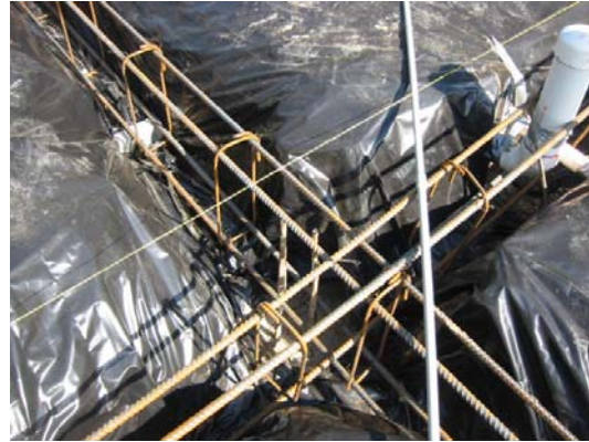
reinforcing steel in a stiffening beam intersection of a slab-on-ground foundation
