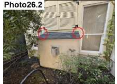
Roof Diverter Flashing Sealants / Seal
