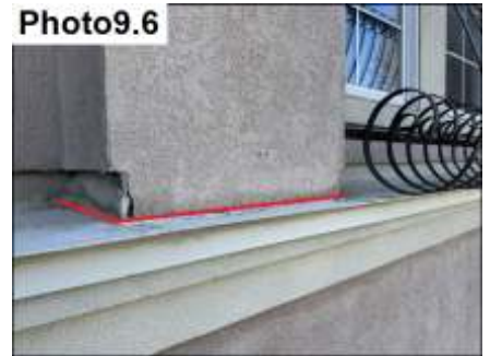
Metal Cap Termination / Seal
