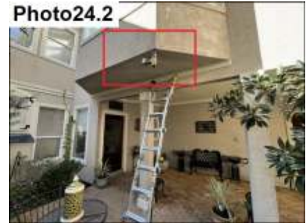
Photo24.2 Substrate Damage / Assess, Repair and Install Proper Relief
