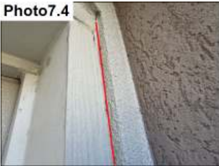
Garage Door Trim Sealant / Seal
