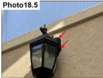
Penetration Sealants / Seal
