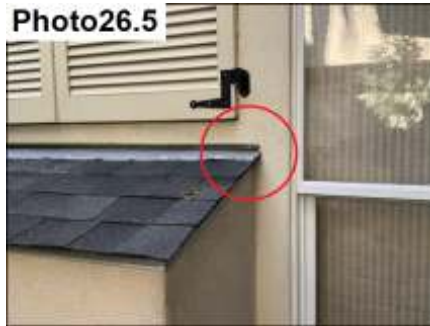
Roof Diverter Flashing Sealants / Seal
