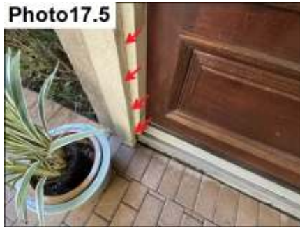
Door Trim and Miter Sealant / Seal
