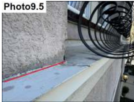
Metal Cap Termination / Seal
