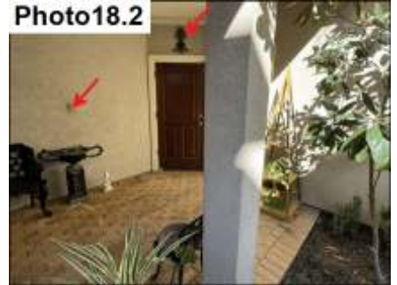
Penetration Sealants / Seal
