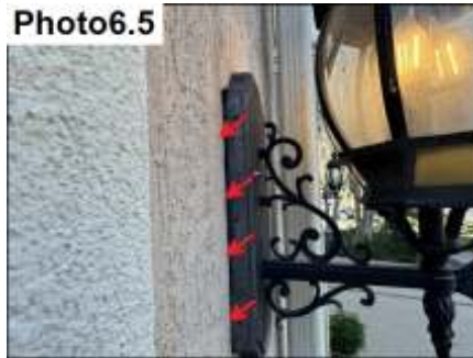
Penetration Sealants / Seal
