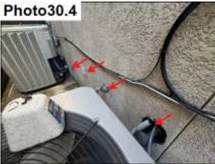
Penetration Sealants / Seal
