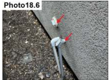
Penetration Sealants / Seal
