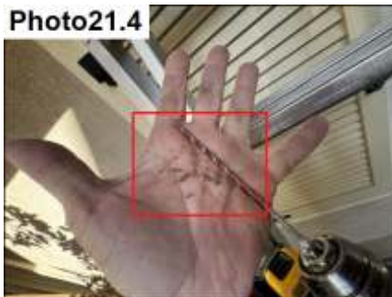
Photo21.4 Substrate Damage / Assess, Repair and Install Proper Relief
