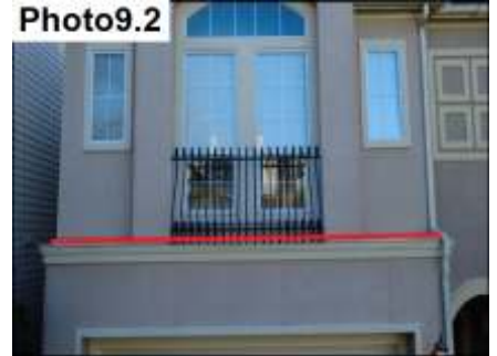
Metal Cap Termination / Seal
