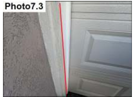
Garage Door Trim Sealant / Seal
