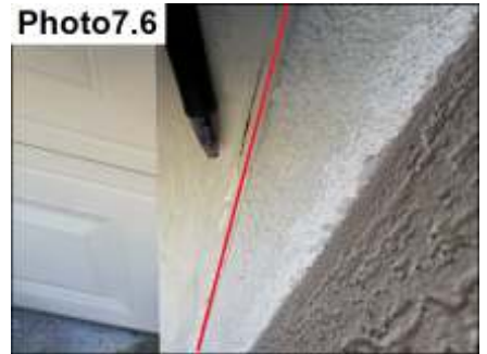
Garage Door Trim Sealant / Seal
