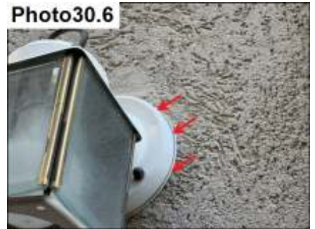
Penetration Sealants / Seal
