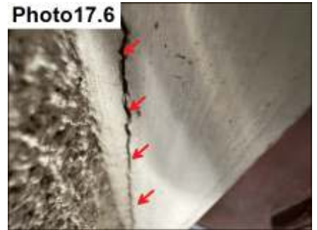
Door Trim and Miter Sealant / Seal
