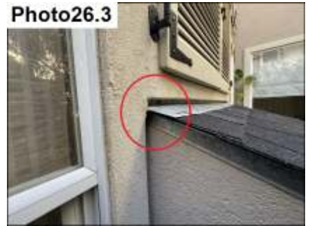
Roof Diverter Flashing Sealants / Seal
