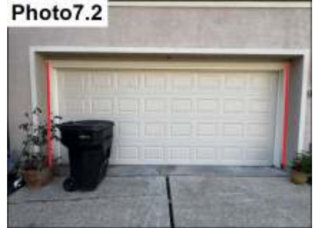
Garage Door Trim Sealant / Seal
