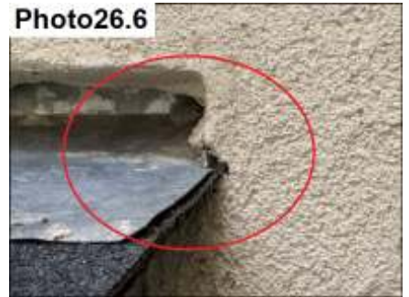
Roof Diverter Flashing Sealants / Seal
