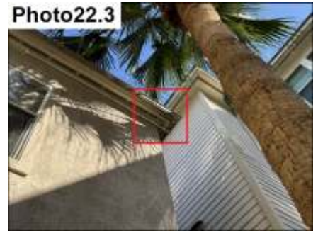
Wood Rot on Fascia / Repair
