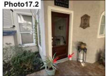
Door Trim and Miter Sealant / Seal
