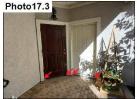
Door Trim and Miter Sealant / Seal
