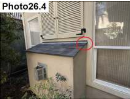
Roof Diverter Flashing Sealants / Seal
