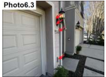
Penetration Sealants / Seal
