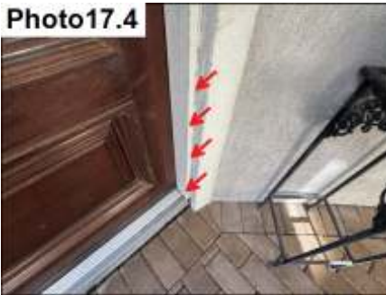
Door Trim and Miter Sealant / Seal
