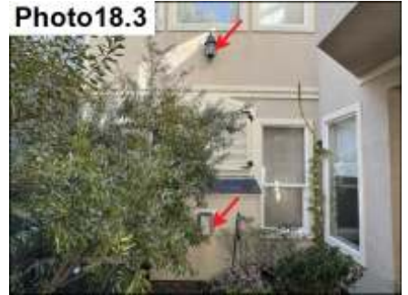
Penetration Sealants / Seal
