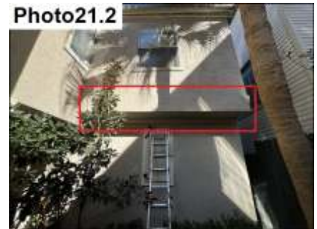
Photo21.2 Substrate Damage / Assess, Repair and Install Proper Relief
