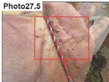
Substrate Damage / Assess & Repair
