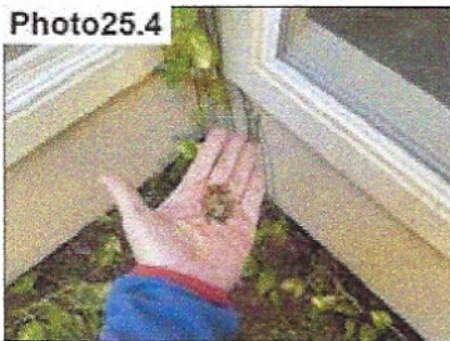
Wood Rot at Bottom Wall/ Repair
