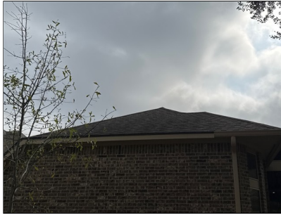
C. Item 14 This roof covering is probably around 5-7 years old and shows signs of wear consistent with its age, except as otherwise noted
