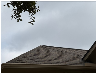
C. Item 15 This roof covering is probably around 5-7 years old and shows signs of wear consistent with its age, except as otherwise noted
