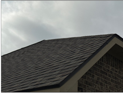
C. Item 13 This roof covering is probably around 5-7 years old and shows signs of wear consistent with its age, except as otherwise noted
