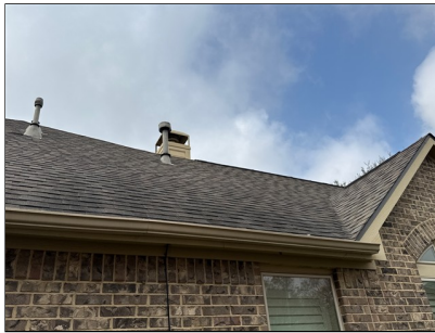
C. Item 10 This roof covering is probably around 5-7 years old and shows signs of wear consistent with its age, except as otherwise noted
