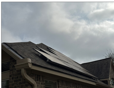
C. Item 18 This roof covering is probably around 5-7 years old and shows signs of wear consistent with its age, except as otherwise noted
