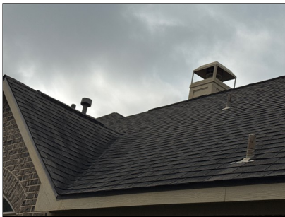
C. Item 11 This roof covering is probably around 5-7 years old and shows signs of wear consistent with its age, except as otherwise noted
