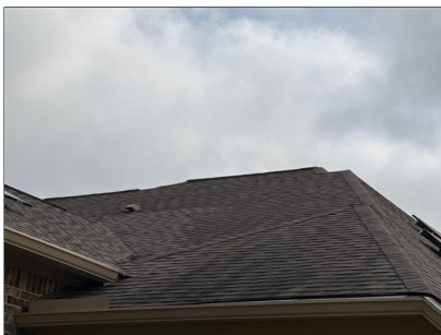
C. Item 17 This roof covering is probably around 5-7 years old and shows signs of wear consistent with its age, except as otherwise noted
