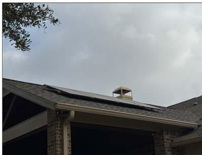
C. Item 16 This roof covering is probably around 5-7 years old and shows signs of wear consistent with its age, except as otherwise noted
