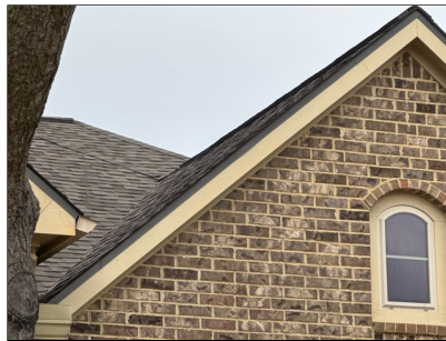
C. Item 6 This roof covering is probably around 5-7 years old and shows signs of wear consistent with its age, except as otherwise noted
