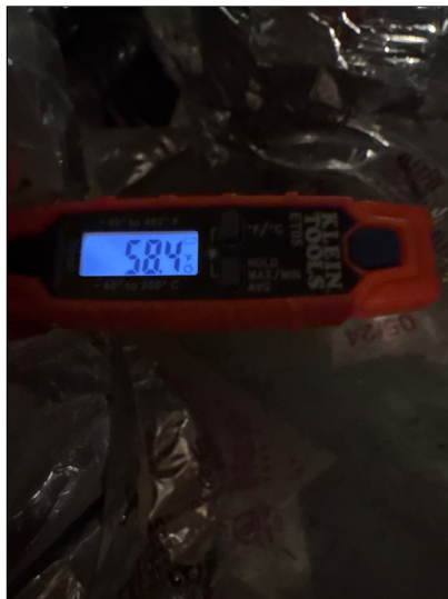
B. Item 2 Supply Side
