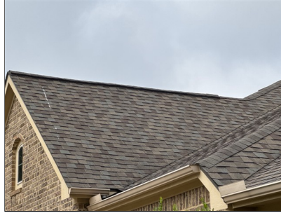
C. Item 2 This roof covering is probably around 5-7 years old and shows signs of wear consistent with its age, except as otherwise noted
