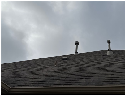
C. Item 9 This roof covering is probably around 5-7 years old and shows signs of wear consistent with its age, except as otherwise noted
