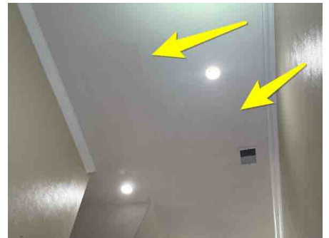
Entry hall, above stairway
