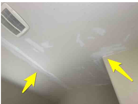
Upstairs left bathroom
