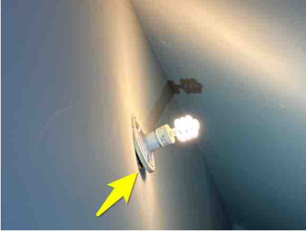
Media room, left attic space/closet
